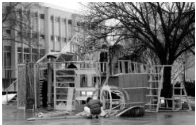
Fig. 2. The individual 4' x 4' x 8' cells being assembled as part of the entire structure.
